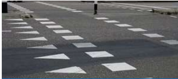
LEFT 47 : Cyclist lane with priority using block markings.
